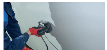
Induktofix® welding disc for AGRU liner
